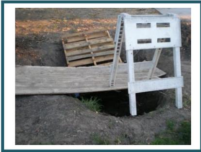
This photo is an example of how **NOT** to set-up a barrier at an excavation.
